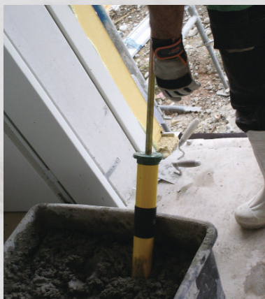
Mörtel in Pumpe saugen
